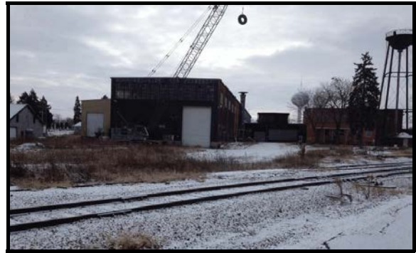
One of the Plymouth assembly buildings
