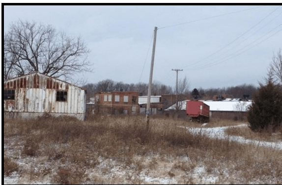
The almost deserted Plymouth Locomotive Works campus in 2016.
